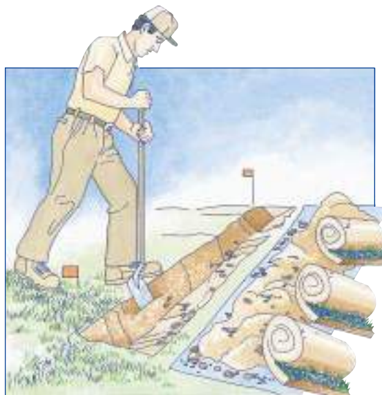
First lay down tarps and remove sod, then dig trenches 10" to 12" deep for the main line. Trench 6" to 8" for lateral lines.
