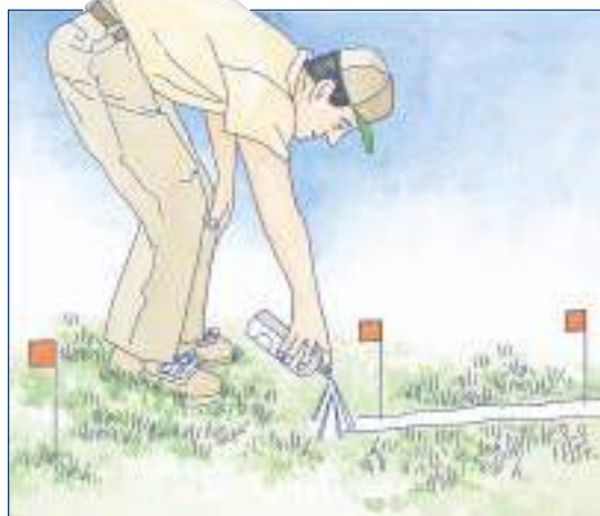
Before trenching, use small flags and marking spray paint to lay out the irrigation system.
