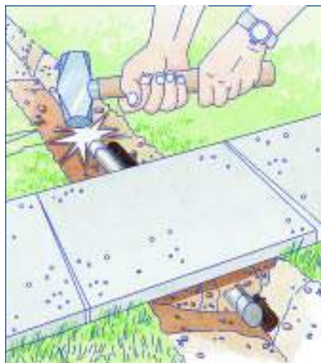
Connect pipe under a walk or driveway by capping off the ends of galvanized pipe and "hammering" through.
